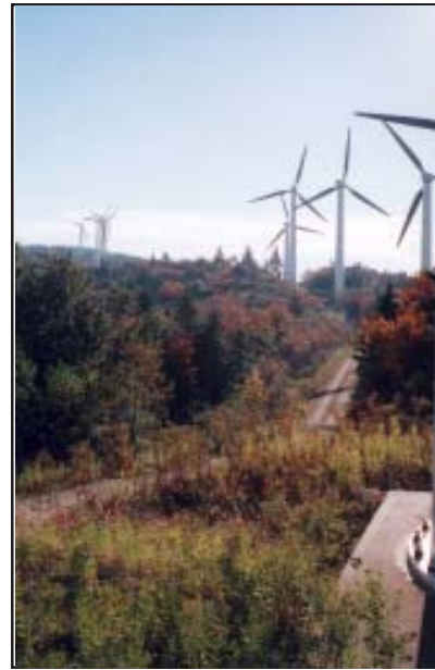
Green Mountain Power Searsburg Wind Facility.
